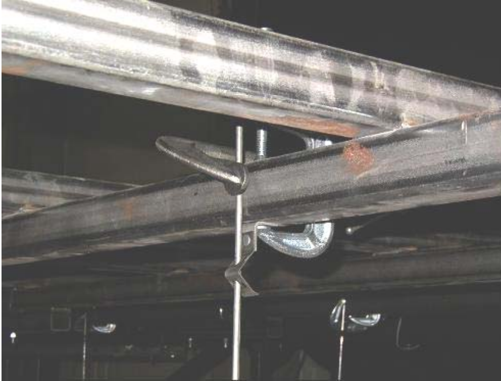
Figure 2–23. C-clamps and top CADDY clip in suspension system 2.
